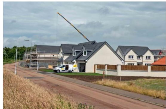
Ground level view with crane in action.
