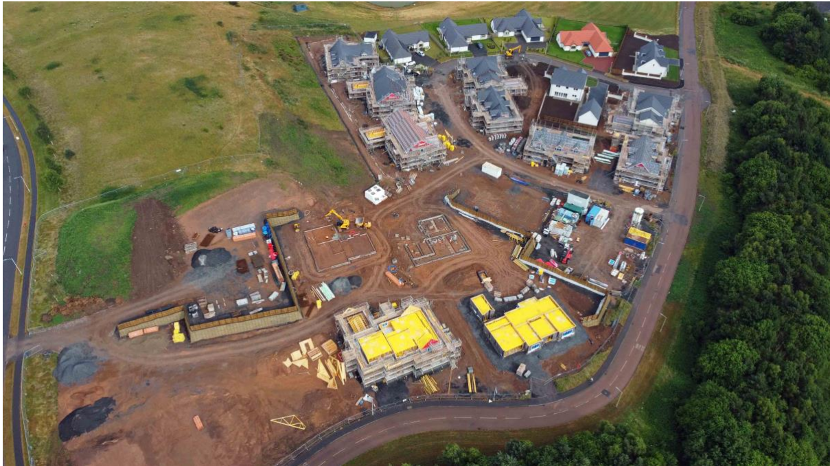
14 houses have been started.
