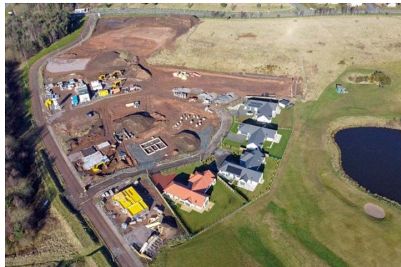
Drone view of the building site.
